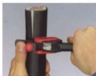
转动工具进行环绕切割 Turning around the cutting tools
